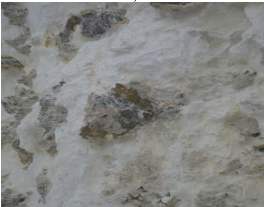
Figure 3. At Nikopol, siliceous inclusions in chawks, Nikopol.
